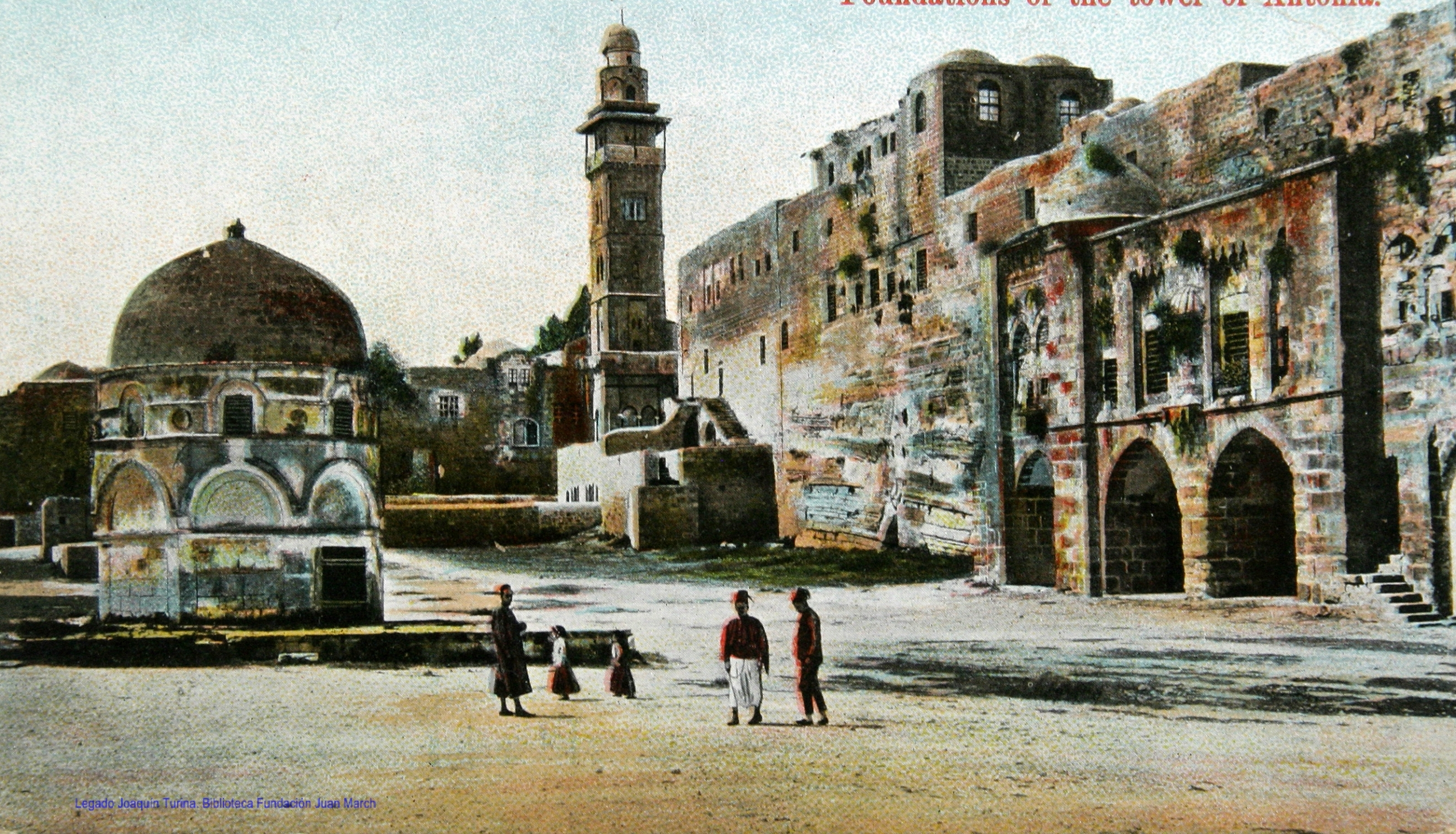
Jerusalem. Platz des Antonia Turms. Assises de la tour Antonia. Foundations of the tower of Antonia.
