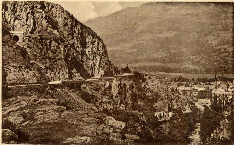
134 CAUTERETS. — ROUTE DE PIERREFITTE À CAUTERETS. — LE GRAND TUNNEL. — LL Legado Joaquín Turina. Biblioteca Fundación Juan March Edit. Gallet. — Cauterets
